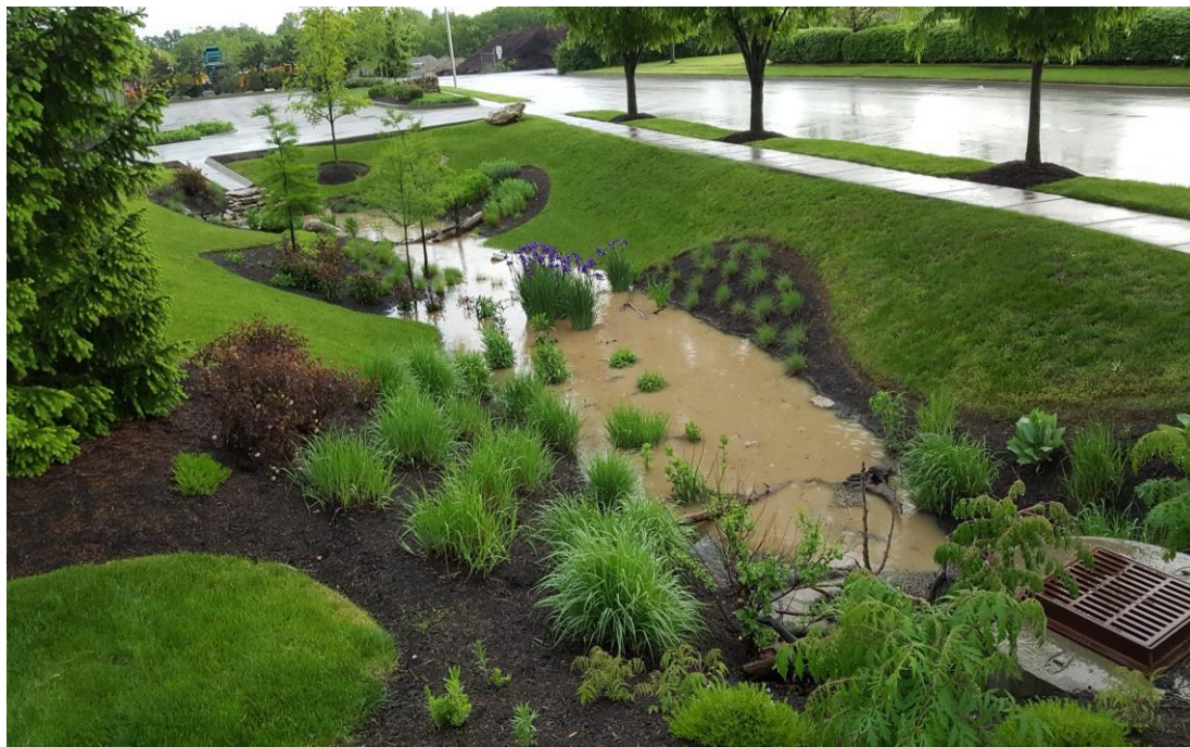
Fig. 3. A residential rain garden planted with deep-rooted perennials — designed to capture rooftop and driveway runoff and recharge groundwater.
